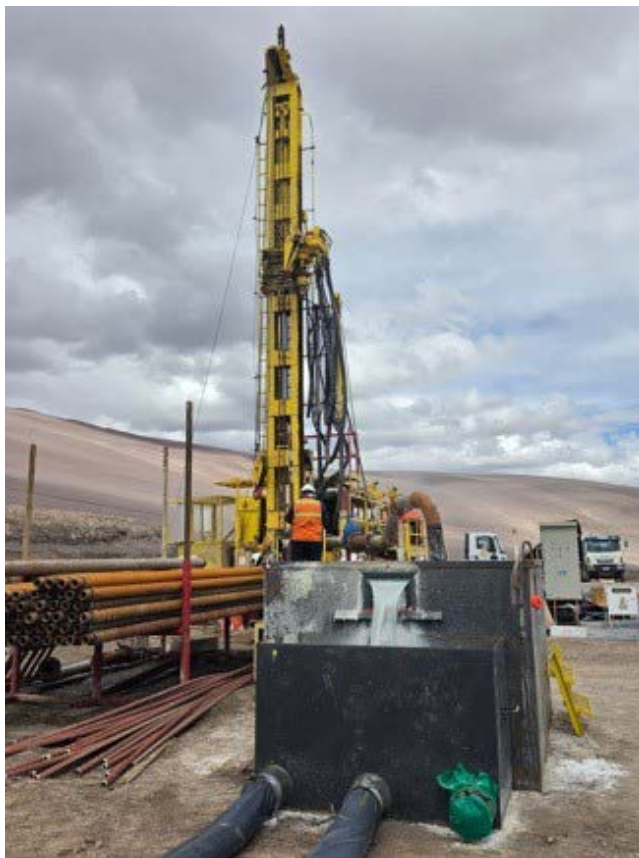
Figure1. Rig at RT-RG26-PW002
