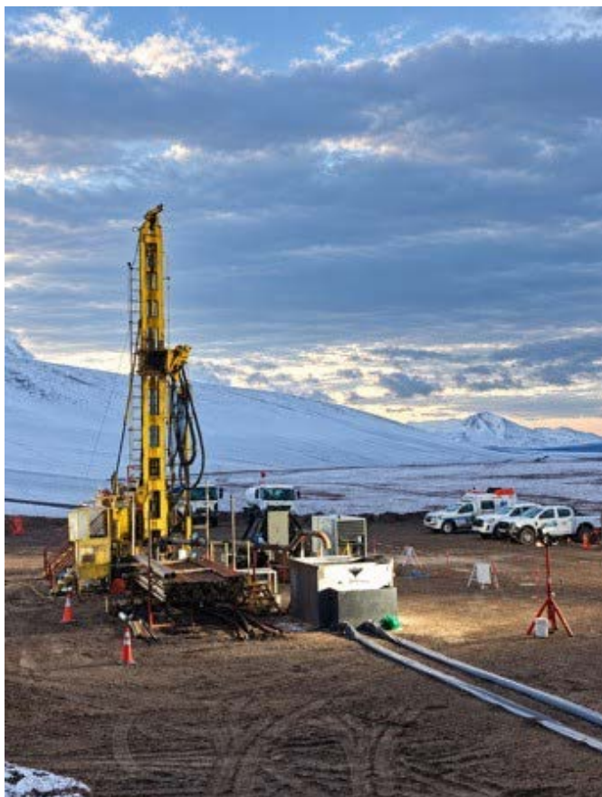
Figure 2. Rig at RT-RG26-PW002
